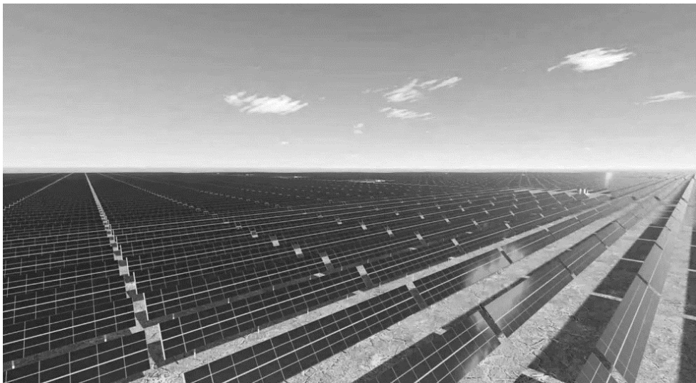
Figura 1. Bhadla Solar Park, 2 245 MW, India
